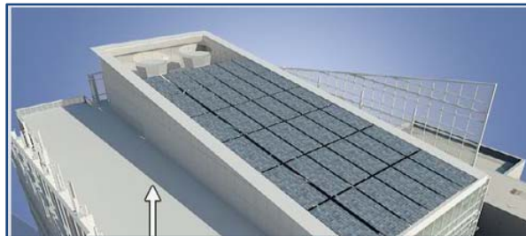
Figure 4: Solar Panels on tower roof
