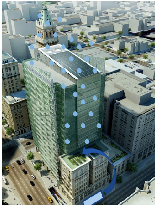
Figure 5: Rain water collection, filtration and reuse system with tank located under the building
