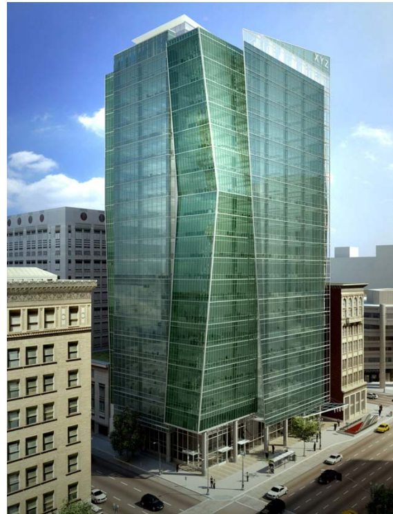
Figure 8: View of the northwest corner of 1100 Broadway
