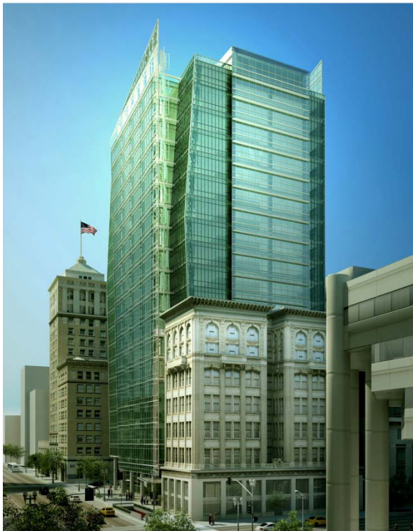
Figure 7: View of the southwest corner of 1100 Broadway
